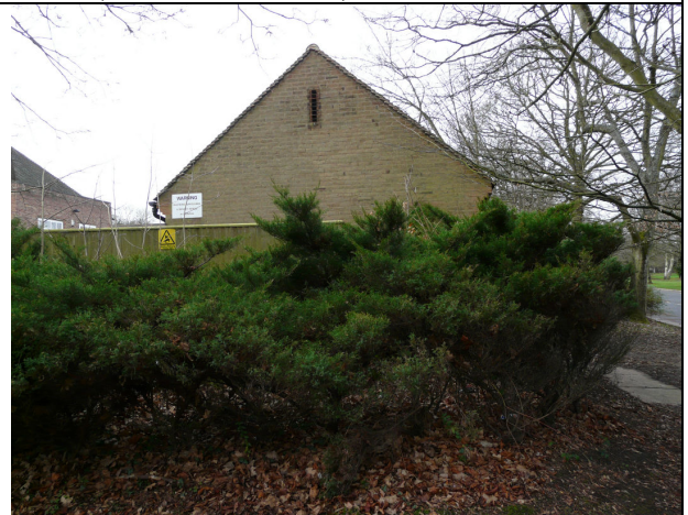
END OF GARAGE BLOCK – NEW GAS MAIN TO EXIT ON END AND RUN IN GROUND AROUND ELECTRICITY SUB- STATION (OPTIONS 1 & 2)
