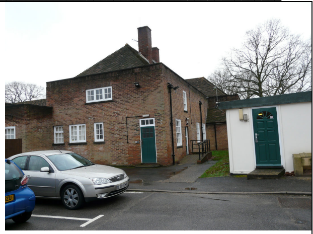
POST ROOM & STAFF RECREATION BUILDING
