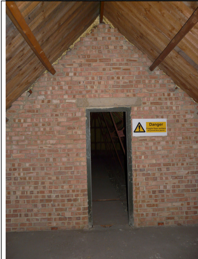
ROOF OVER DINING ROOM – SECTION WITH NO ASBESTOS SHEETING
