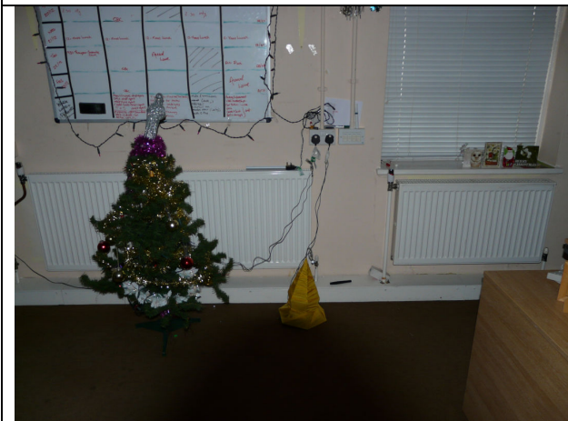
EXISTING PIPEWORK AT LOW LEVEL IN PIPE CASING
