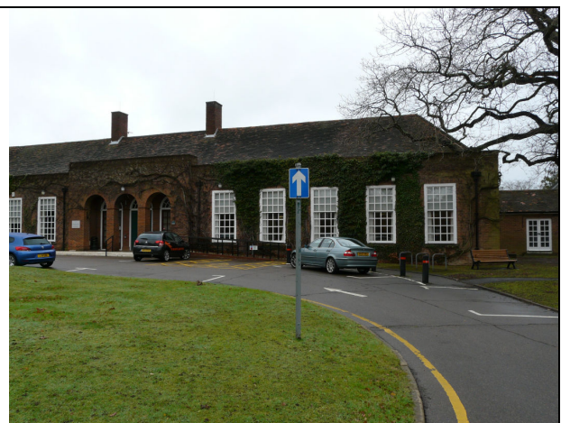
CENTRE AREA – COUNCIL CHAMBER & ENTRANCE
